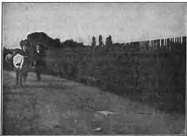
FIG. 215.—German fence made of forest thinnings. Uprights are first thinning 1\frac{1}{2} – 2\frac{1}{2} inches in diameter, round. Cross pieces are second thinning split. Posts are larger round pieces. No saw dust or slab waste. The forest was planted with trees about as far apart as hills of corn in American field.
